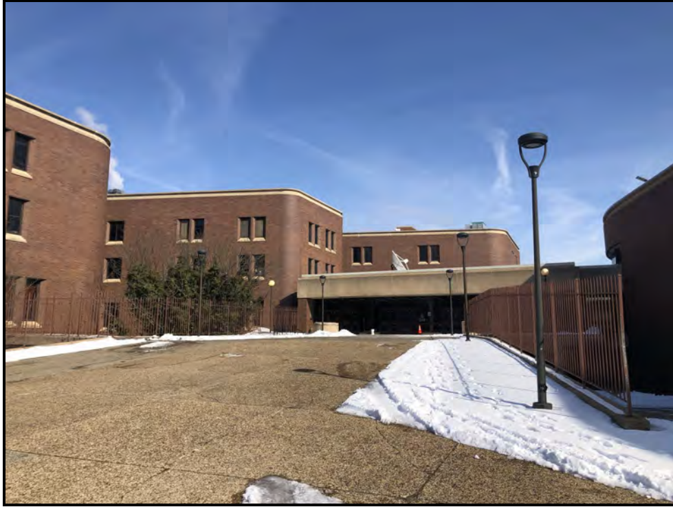
Photograph 1: View of the western portion of the high school structure.
