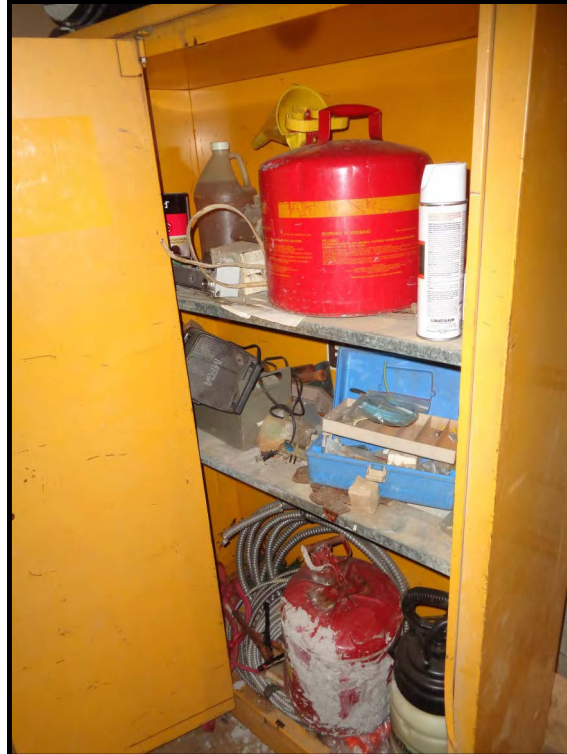
Photograph 11: View of a fire cabinet with two (2) 5-gallon gas cans.
