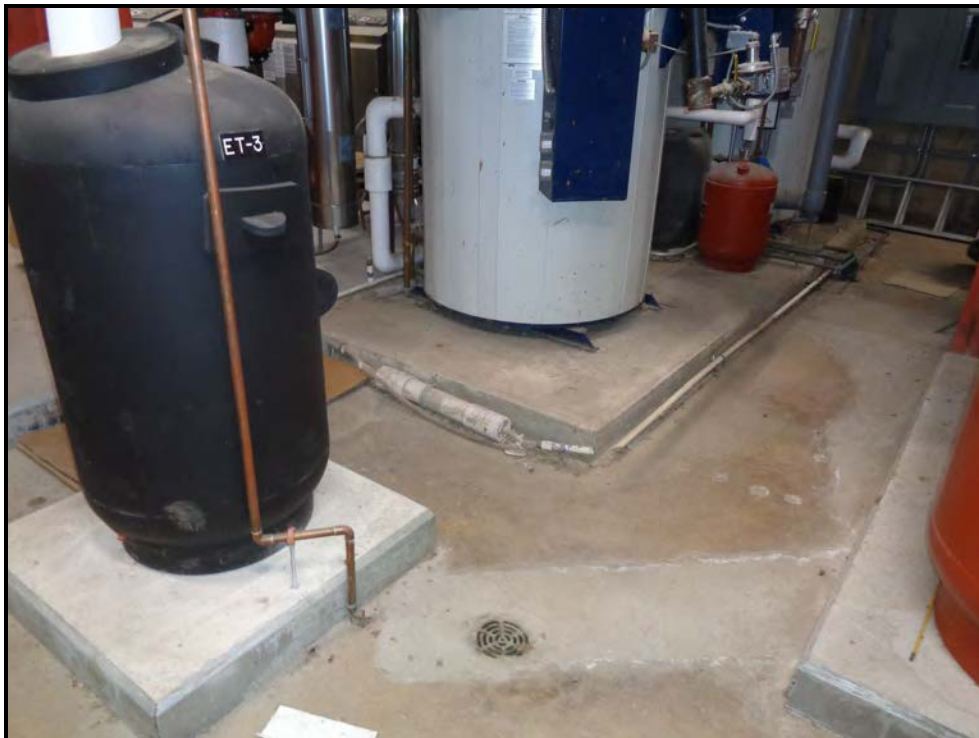
Photograph 13: View of a floor drain within the maintenance area of the high school.
