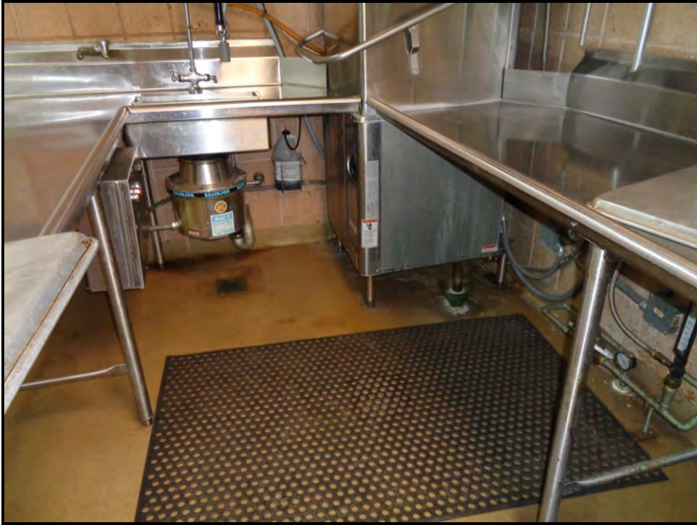
Photograph 18: View of floor drains within the kitchen area of the high school.
