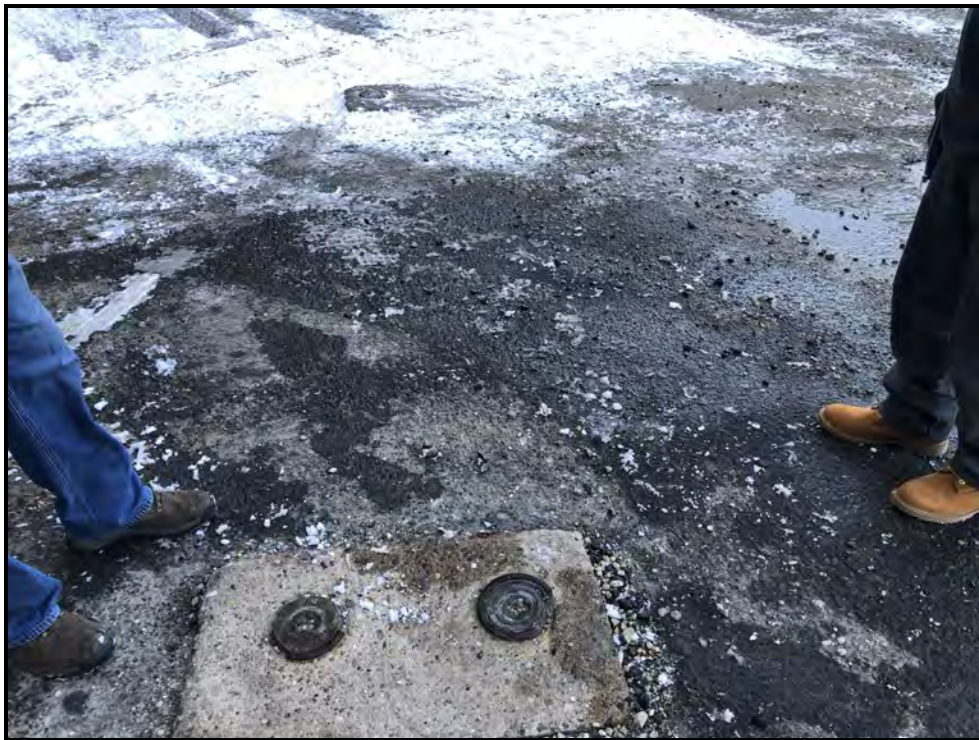
Photograph 9: View of four (4) UST fill ports located at the north of the high school structure.
