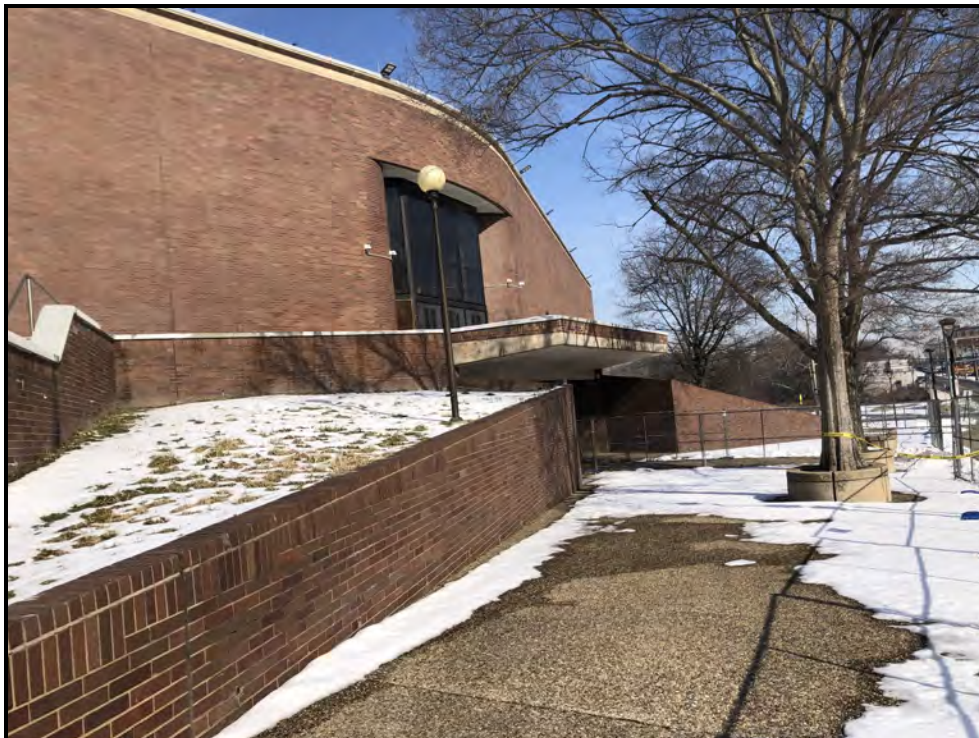
Photograph 2: View of the southern portion of the high school structure.
