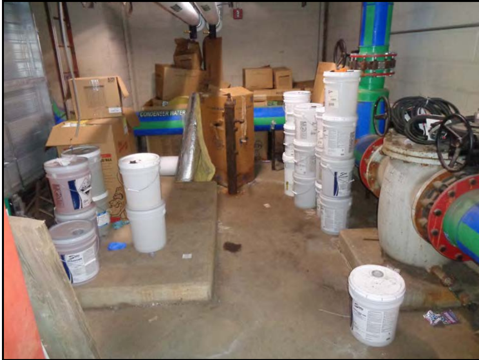
Photograph 10: View of twenty-one (21) 5-gallon buckets including algacides and corrosion inhibitors used for hot water heaters located within the maintenance area of the high school.
