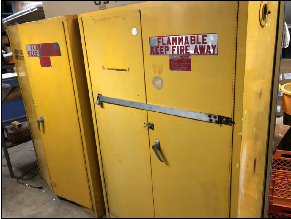
Photograph 14: View of two (2) fire cabinets (one with storage boxes/one locked).
