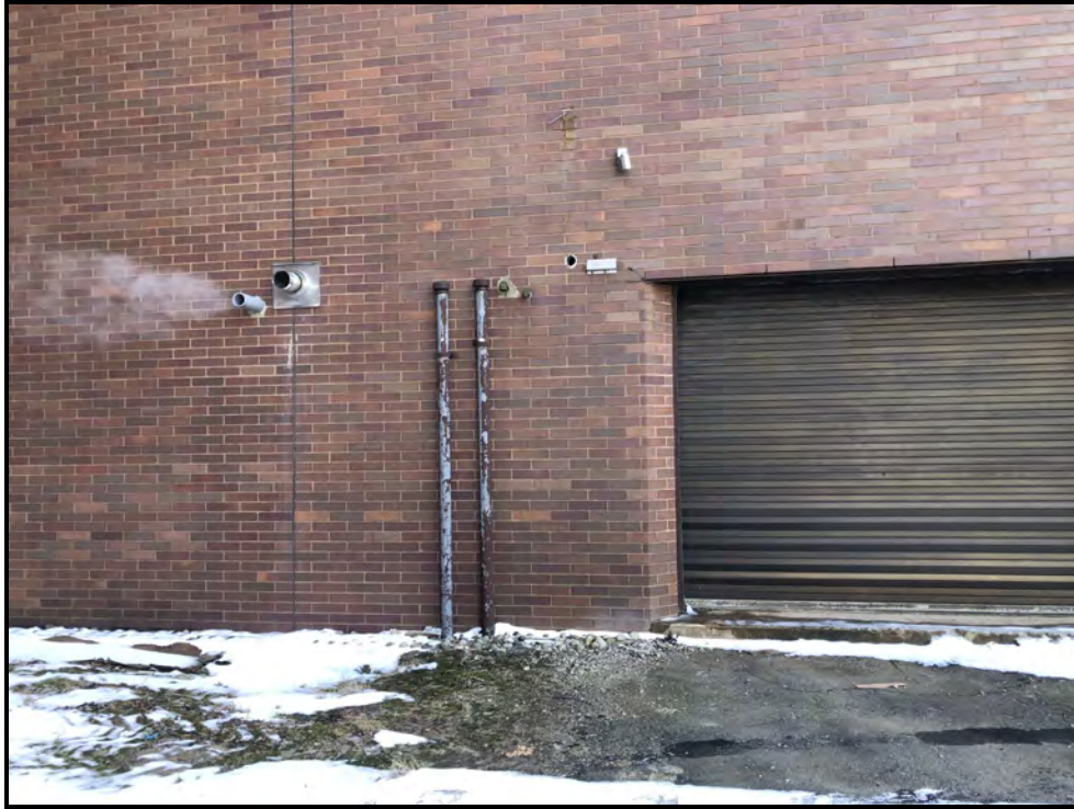
Photograph 8: View of two (2) UST vent pipes located at the north of the high school structure.
