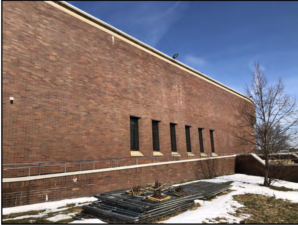
Photograph 3: View of the northern portion of the high school structure.
