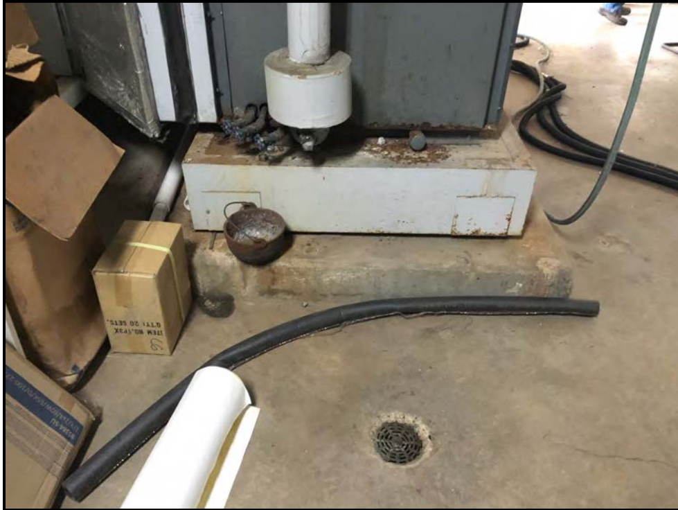
Photograph 12: View of a floor drain within the maintenance area of the high school.
